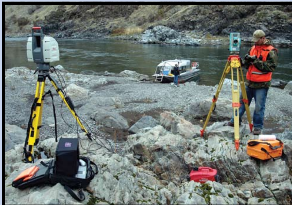
A Glahe & Associates field technician ties into a local control network with a reflectorless total station while Idaho Power employees help set up laser scanner targets.
