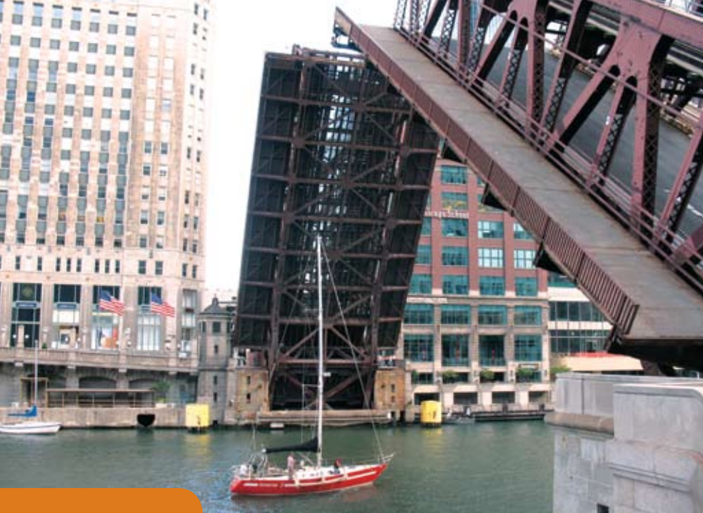
Above: The bridge's fixed-trunnion design allows its leaves to be raised and lowered to accommodate boat traffic on the Chicago River. Below: An orthophoto and line work of a bridge house.
